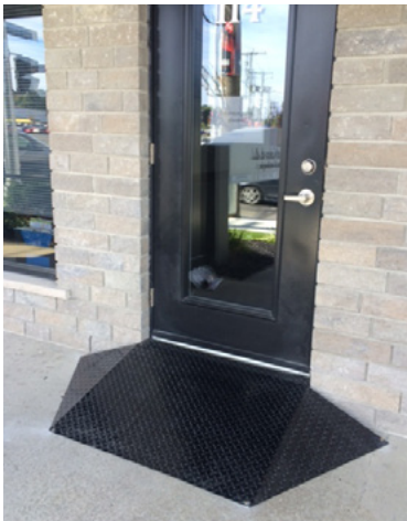
Descente handicapés- Disabled ramp
