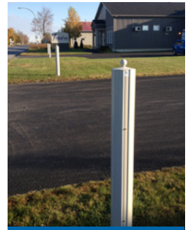
Bollards B-6 Bollards
