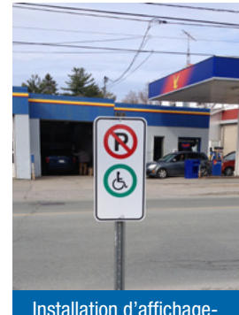
Installation d'affichage- Signs installation.
